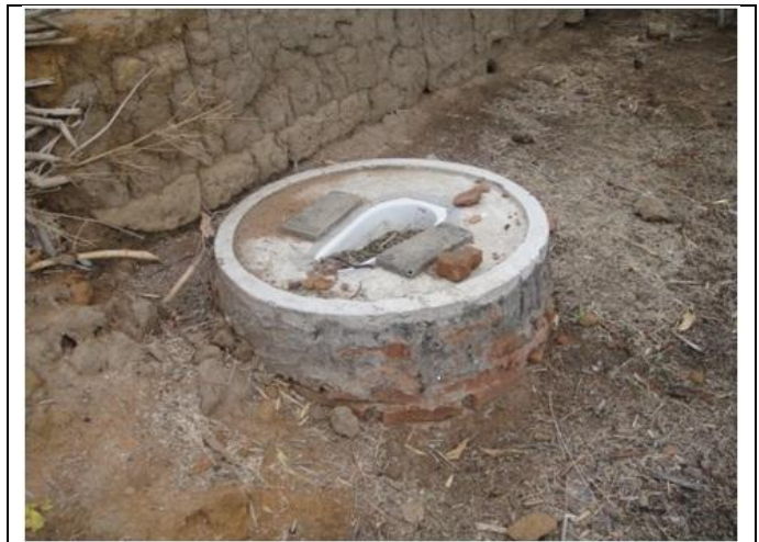
Figure-1: Photograph showing no super structure (Anuppur/NGP)
